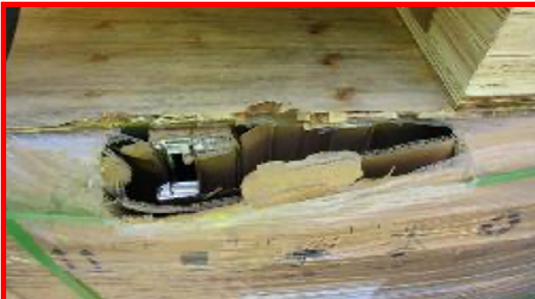
Pallet wear and tear or damaged modules
